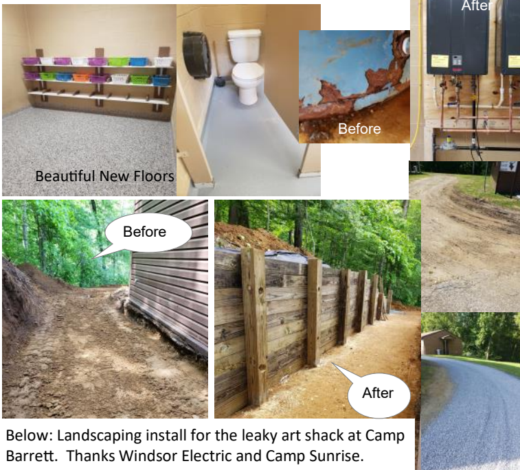
Below: Improvements at Camp Barrett
